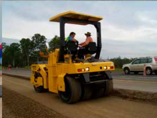
Soil subbase, Australia
