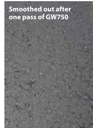
Fig 4. Remove hairline cracks from HMA pavement
