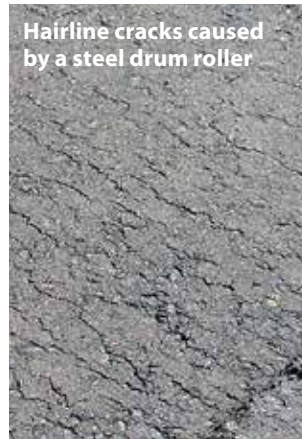
Fig 4. Remove hairline cracks from HMA pavement
