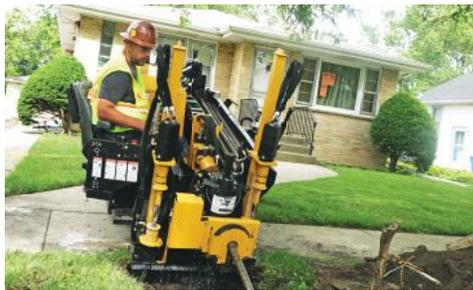
**MORE POWER.** Equipped with a 48 hp (35.8 kW) Kohler engine, this drill offers 1200 ft-lb (1627 Nm) of spindle torque and 7850 lb (3563.9 kg) of thrust/pullback.
